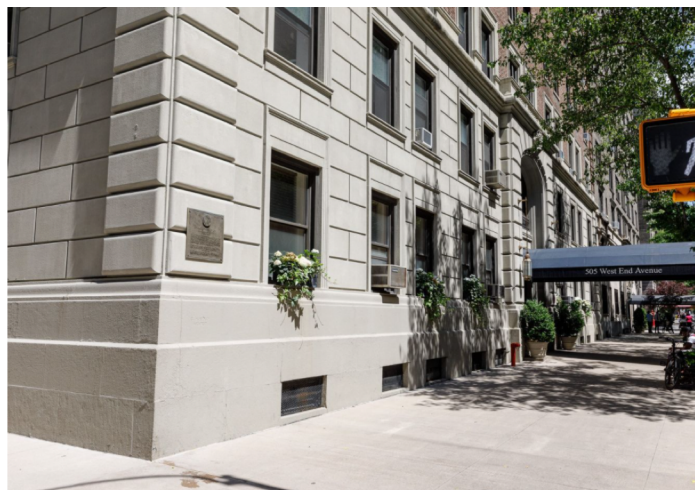
The exterior of 505 West End Ave., a pre-war building on Manhattan's Upper West Side, where Praneet Gill combined two co-op units.
